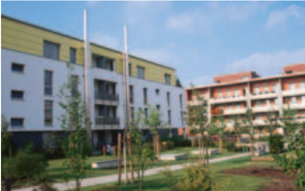
GETEC mbH heating centre location
