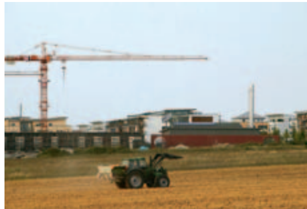
Comprehensive school under construction
