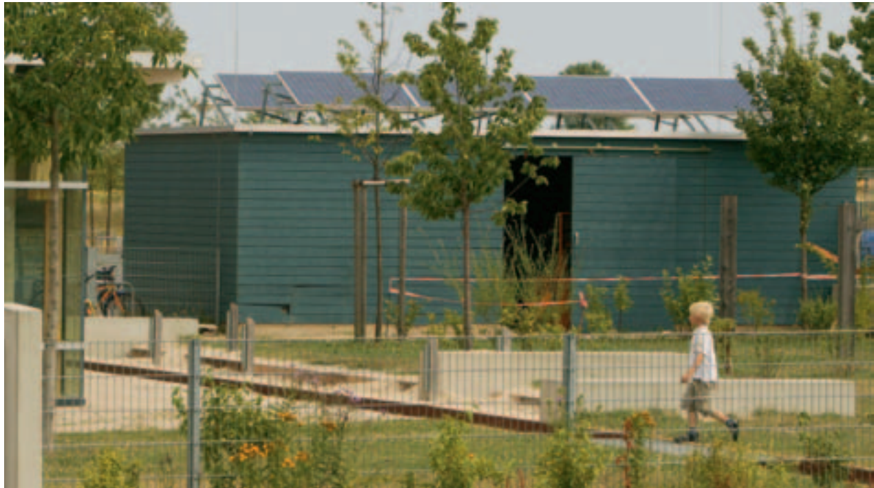
Photovoltaic installation at Kronsberg primary school
