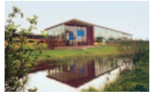
Rainwater retention pond at the primary school
