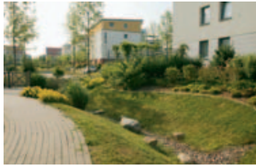
Hollow and trench drainage system
