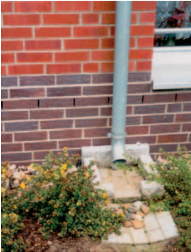
Drainpipes and gullies
