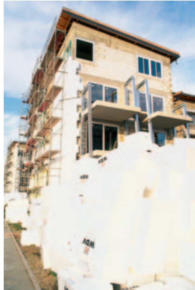
Insulation during construction
