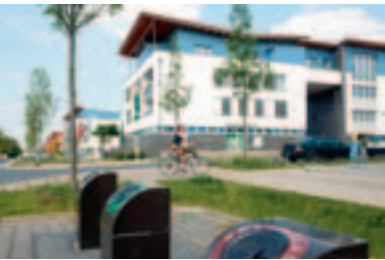
Underground bottle banks
