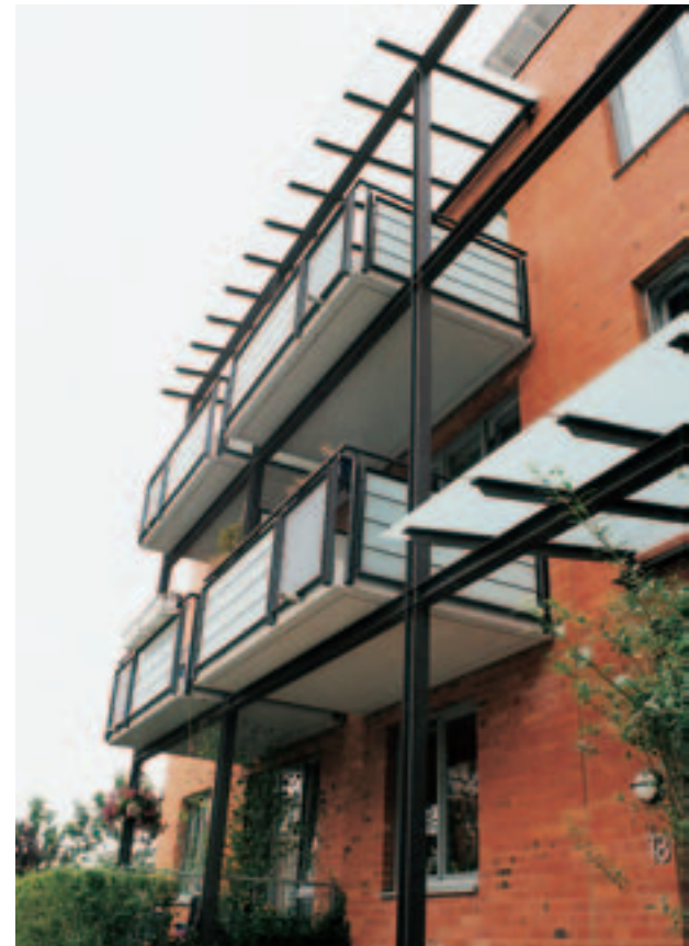
Balcony floors thermally separated from the façade
