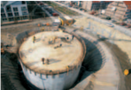
Thermal storage tank under construction
