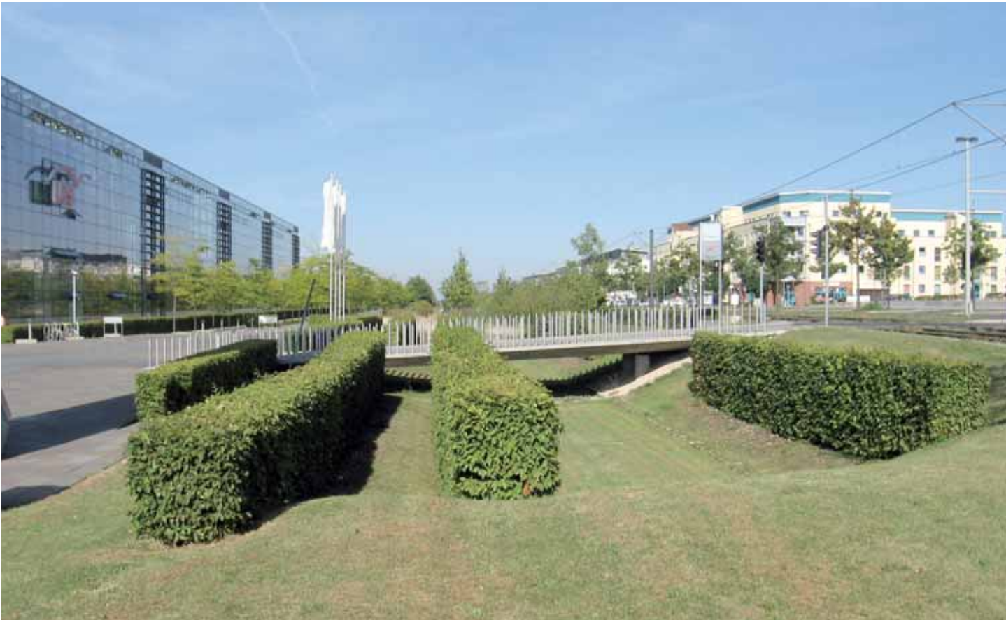
Retention am Hangfuß | Rainwater retention at the foot of Kronsberg hill
