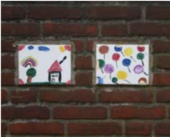
Detail Mauer, Wilhelm-Schade-Schule
